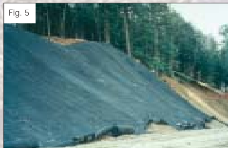
After installation and before vegetation
