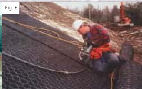
Adjacent MacMat® R panels connected using 'hog rings'
